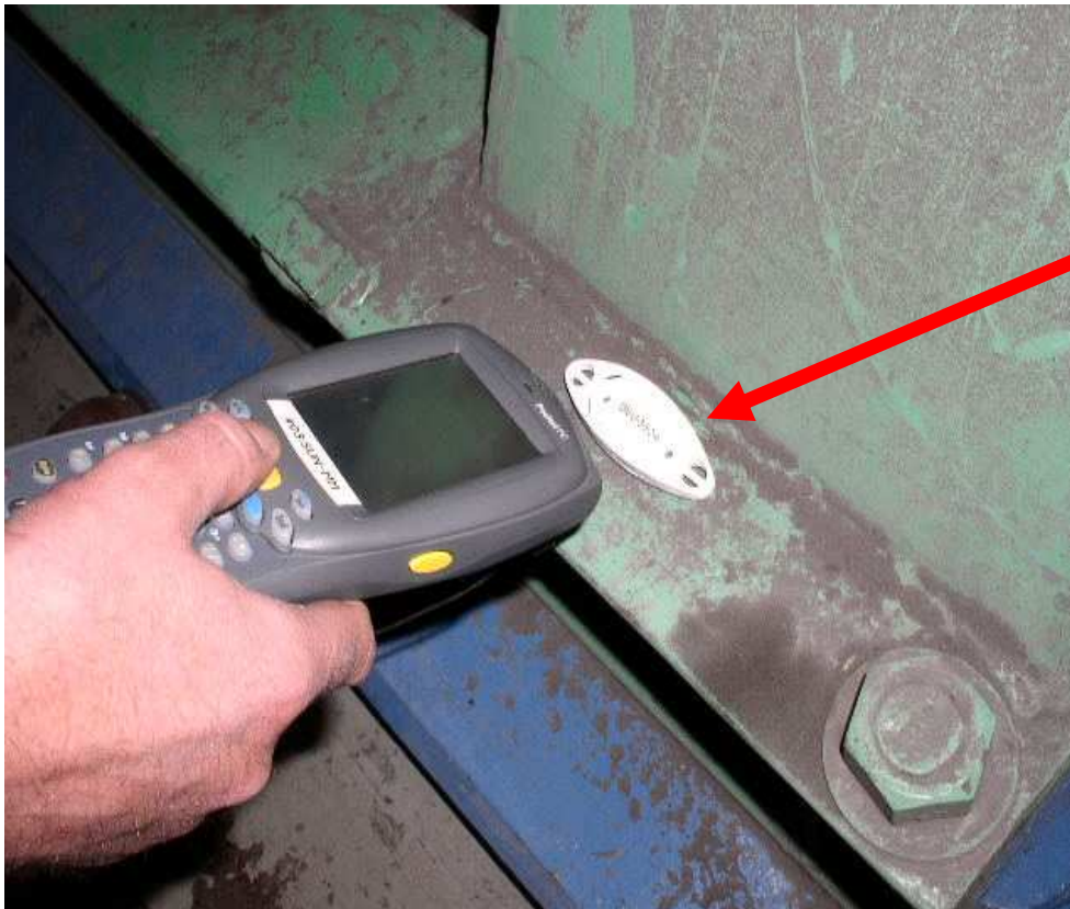
RFID Tag Mounted on Equipment
